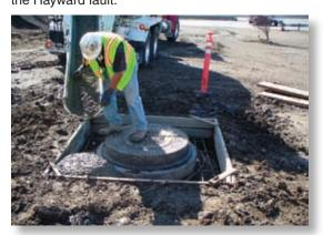
From the top: Pipe casings up to 60 inches were used to create a new crossing; A tunnel boring machine was used to excavate under I-880; New manholes were set to access the new sewer pipes.
