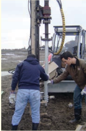
Ground screws being tested
