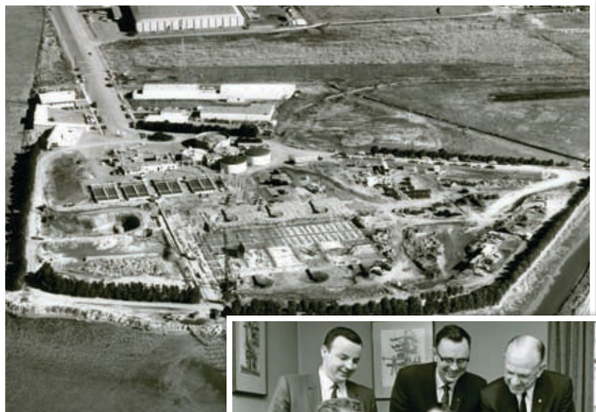
Above: New treatment plant under construction in 1967.
